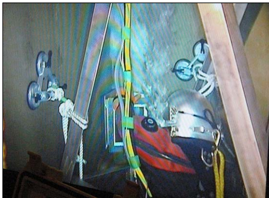
Diver conducting vacuum box test in IP2 spent fuel pool.
